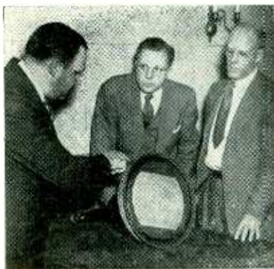
Single-gun three-color picture tube, which is expected to hasten the realization of color television
